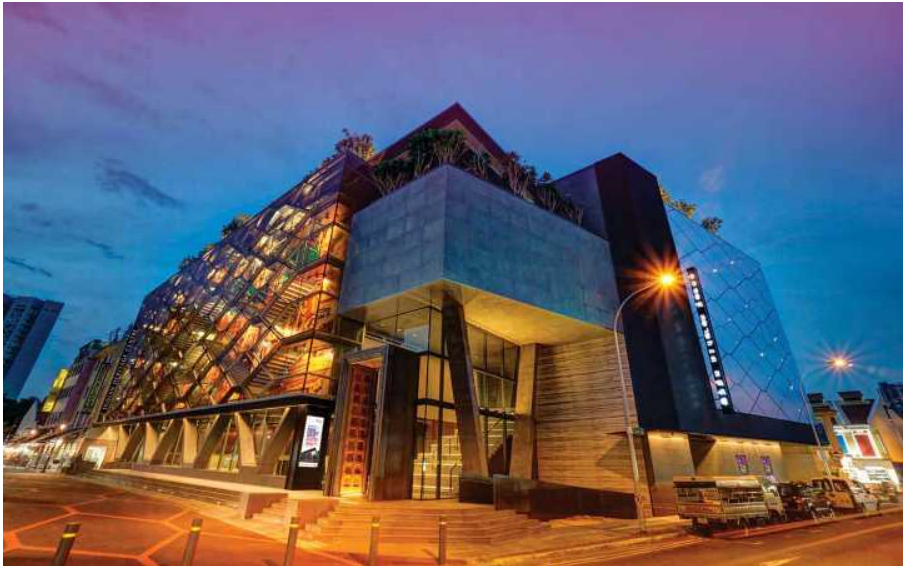
Figure 2. The Indian Heritage Centre (IHC). Image courtesy of IHC.
